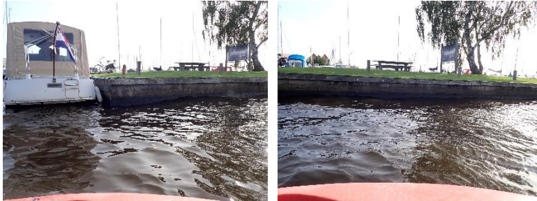
Sheet pile of okan
