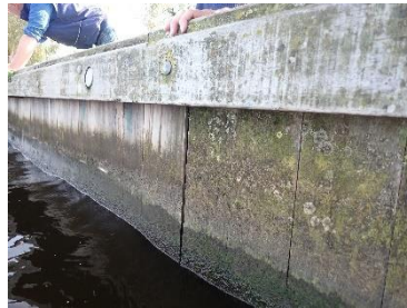
Transition of the angelim vermelho -larch sheet piling to sheet pile 1a okan
