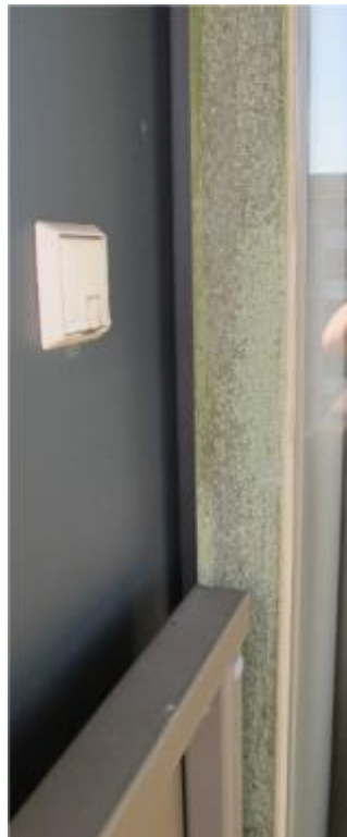
Figure 14: Unpainted joinery with lichen on moisture areas.
