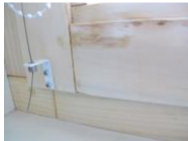
Figure 16: Clean inside timber surface with some brown discolorations.
