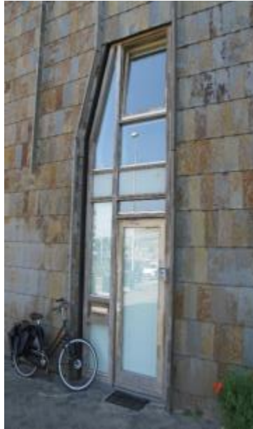
Figure 13: Unpainted joinery, clean, partly homogeneous discoloured, partly heterogeneous e.g. door.
