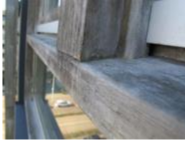
Figure 17: Clean and homogeneous discoloration (greying).
