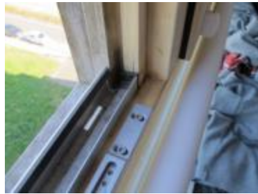
Figure 18: Clean joinery and non-corroded locks.
