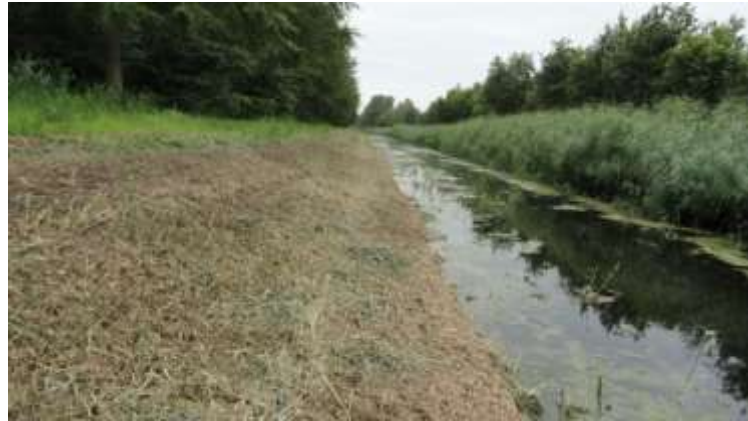
Figure 2: Fresh water test (canal lining) in the Netherlands (wood sheets installed on left and right position of the water way).
